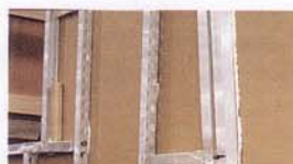
Each sidewall is constructed for strength and is heavily insulated for comfort. The inside consists of 5/8" of beaded foam, laminated to kraft paper and covered by interior paneling. Outside, the
