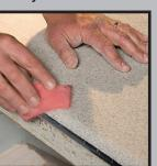
sanded, custom-fitted and seamlessly integrated with backsplashes and in-line sinks to create a single surface with no cracks for easy clean-up. They are non-porous, and heat and scratch resistant. Newmar craftsmen expertly fit, finish and install them.
